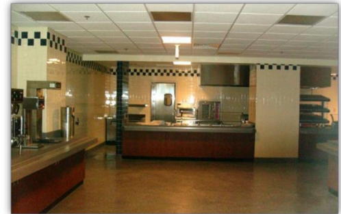
GSA Federal Building Cafeteria Interior Renovations Richmond, VA
