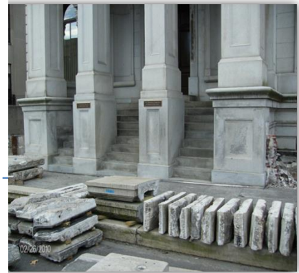
Lewis F Powell Courthouse Structural Repairs Richmond, VA
